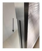
Turn foot bar upside down and slide first bar into the channel on the side of the panel. Do this from the top, sliding the bar all the way down.
